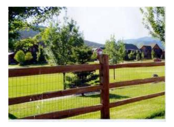
Three Rail Split Rail Fence with optional wire mesh.
